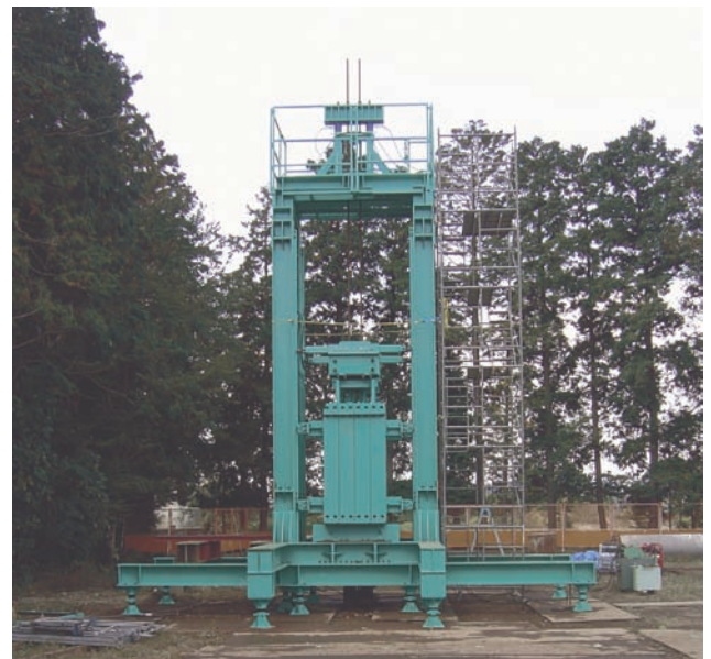
Figure 4. Rapid load test of cylinder pile using a 432 kN cushioned drop-mass system.
